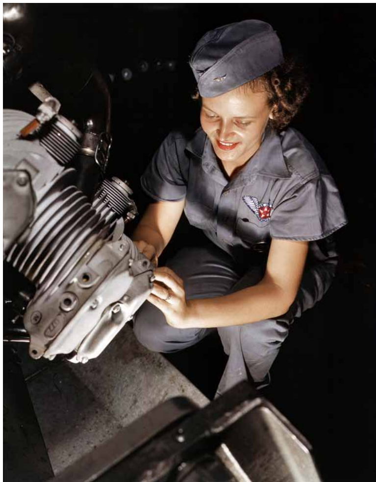
TOP LEFT: "August 1942. Mechanic Mary Josephine Farley works on a Wright Whirlwind motor in the Corpus Christi, Texas, Naval Air Base assembly and repairs shop. 4x5 Kodachrome transparency by Howard R. Hollem."
